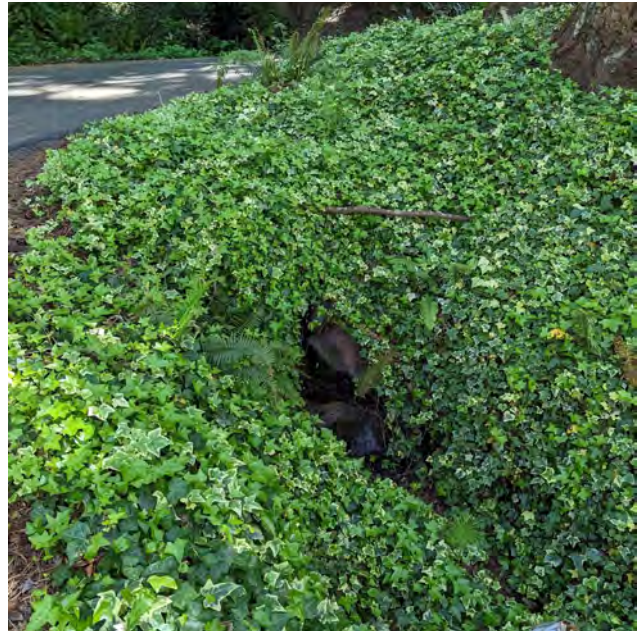
Upper segment of culvert under driveway
